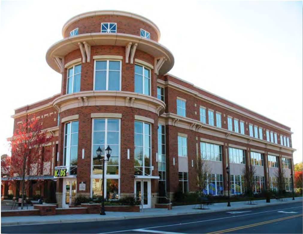
Huntersville’s Town Center, which includes a children’s museum as well as Town offices, was completed in 2010 and is one-quarter mile from the LYNX Red Line station.
